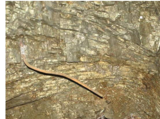
Spalling and crushing
