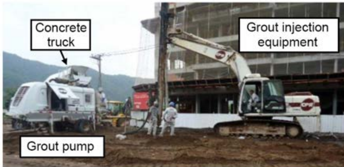
Figure 2. Grouting work in progress at Pontal Oceânico.
