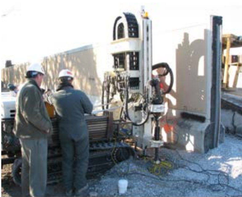
Figure 3: Geoprobe CPT rig at Levee Concrete Wall on Sheet Pile
