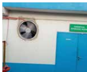
Installation of Extractor at Chemical store
