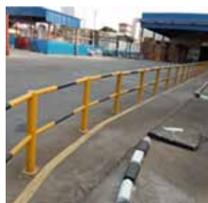
Installation of safety barrier at entrance to FG WH
