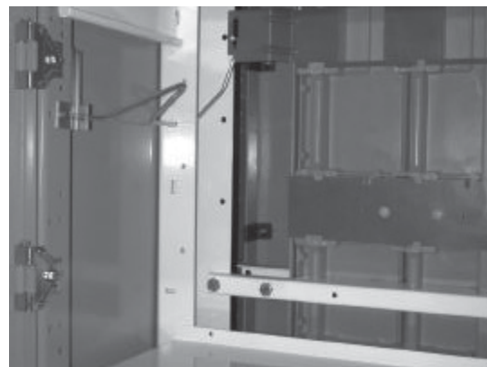
Figure 34. Shutter arm linkage
