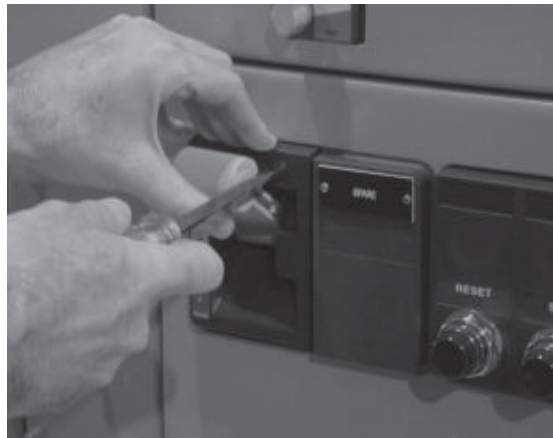
Figure 36. Defeater mechanism
