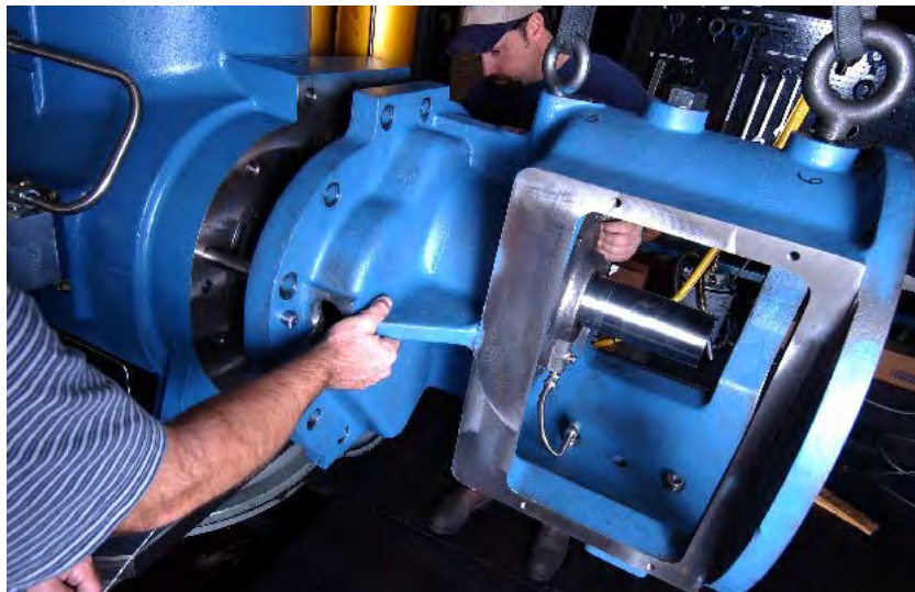
Figure 5-25: Re-Installing Gearbox on Compressor
