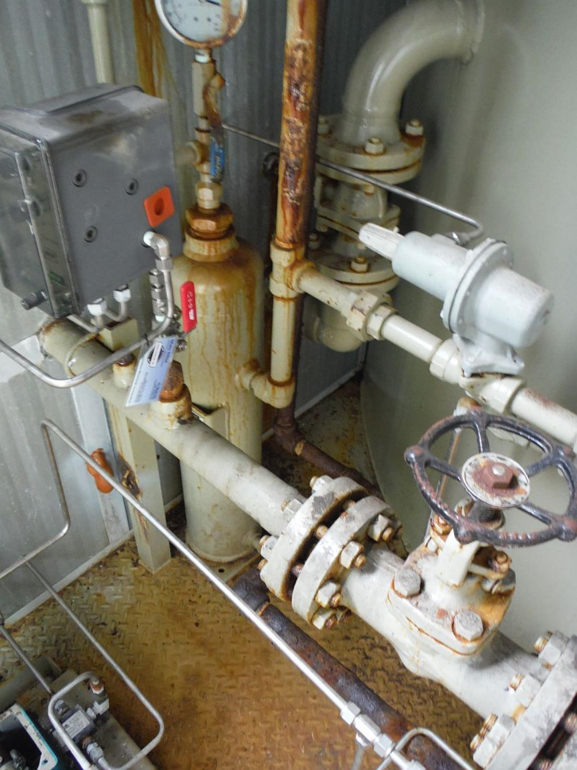
UVL ID#: 16853F S N: S5573-14 Man: WELLMARK Set Press: 150 PSI Model: W9501-RSA 200 Capacity: 433 SCFM Cold Diff: Back Press: Size: 1 " MNPT X 1"FNPT A#: N/A Vessel SN: N/A WO#: 306710 PO#: N/A PO Line# N/A REVISION 2 55
