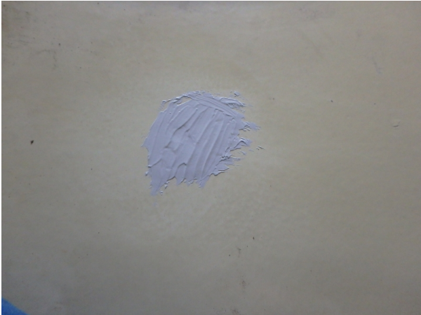
Photo 3: Coating Chip Repaired
