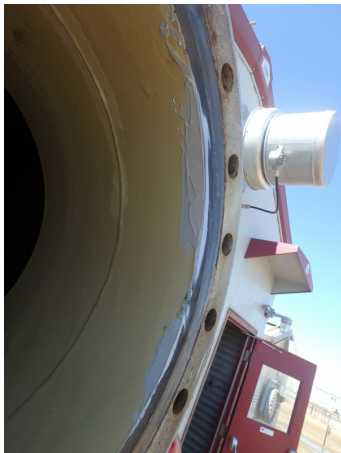
Photo 5: Manway Coating Repaired
