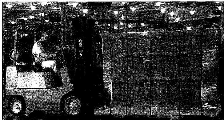
Figure 2: Moving the MCC with a Fork Truck
