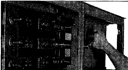
Figure 34: Removing the Bolts from the Splice Assembly
