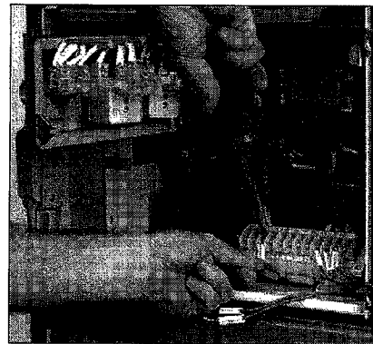
Figure 95: Connecting Control Leads to the Terminal Blocks
