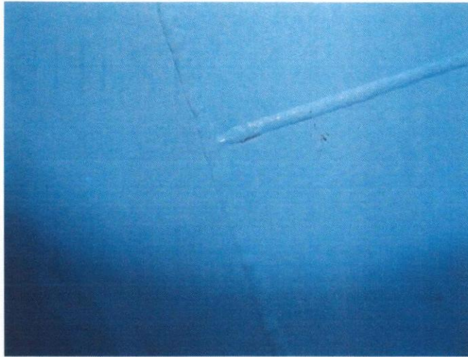
Typical as new coating of a Tee Seam
