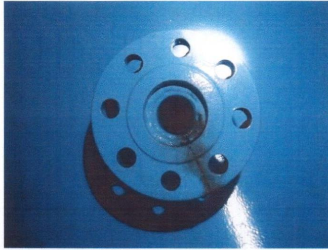
internally flanged nozzle with As new condition coating
