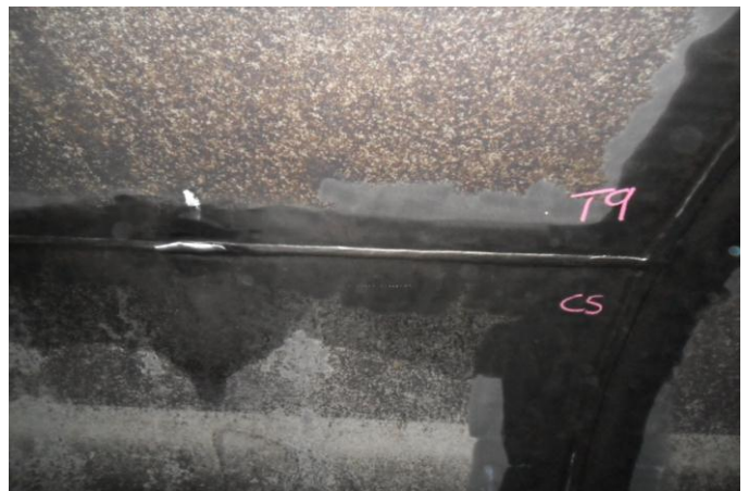
C5 / T9 Indication in Start / Stop 24" West of C5
