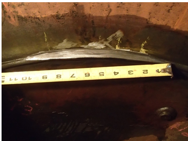
Photo 3: West Head Weld Repair
