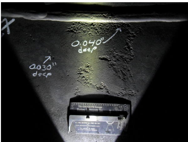
Photo 7: Corrosion on East End (2)
