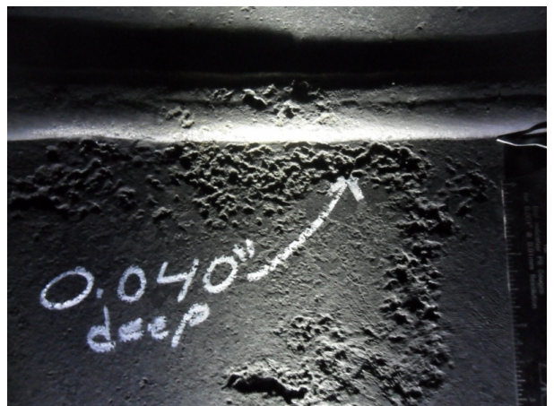
Photo 8: Corrosion on East End (3)
