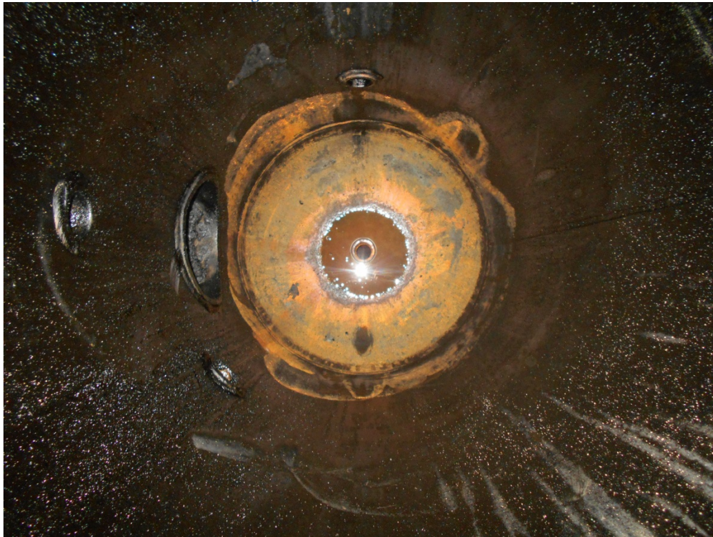
Figure 10 Looking Down Into The Boot
