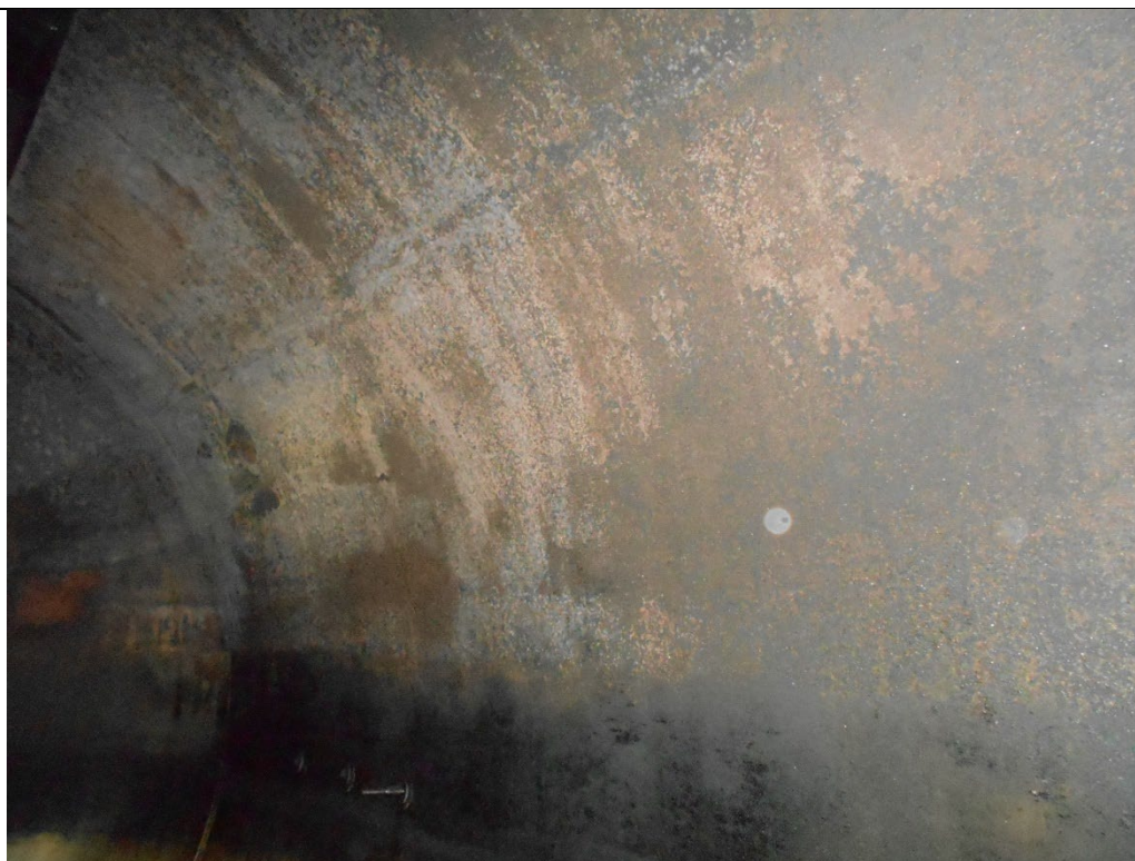
Figure 15 3rd Stage Uncoated Wall
