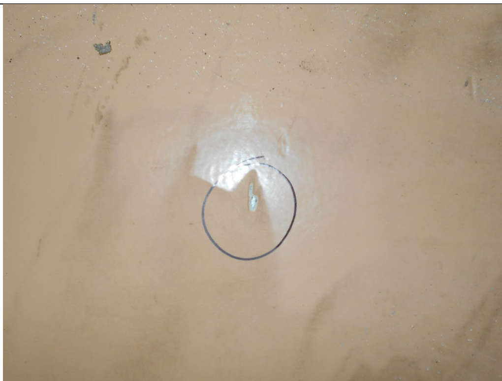
Figure 5 Example of Chip in Coating
