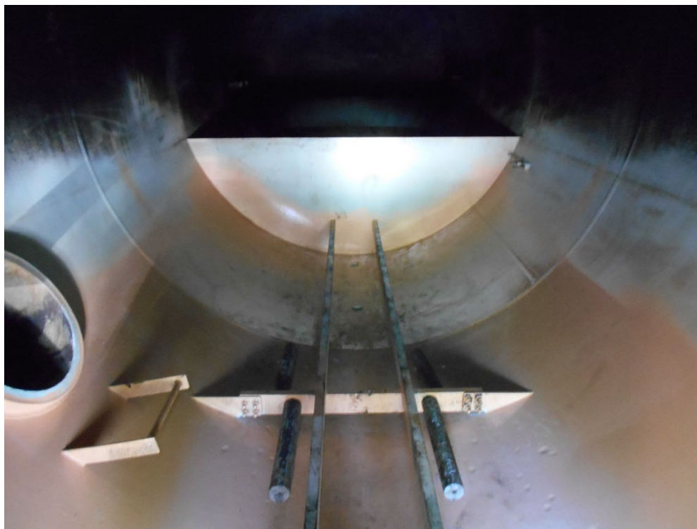
Figure 2 Anodes and 3 rd Stage Weir near Manway
