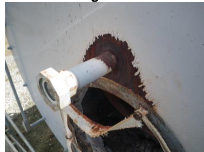
8) Previous Hot Gas fugitive emission on manway:
