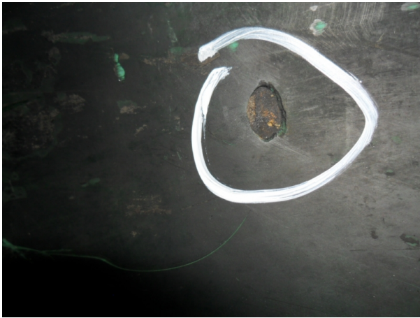
Photo 5: Coating Chipped (2)
