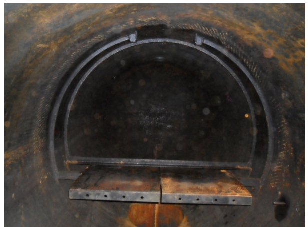
Photo 8: New Demister (In Behind The Front Screen)
