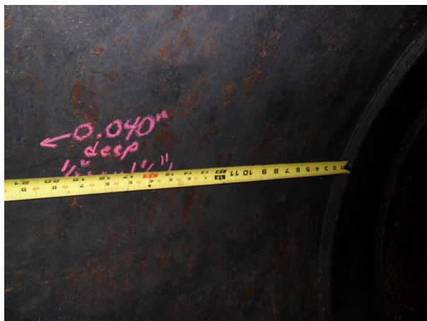
Photo 21: Pitting and Mechanical Gauges (5)
