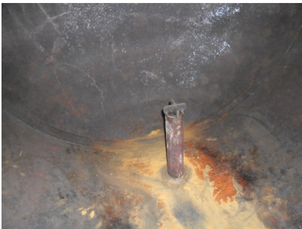
Photo 11: Vortex Breaker in Can 2 North End
