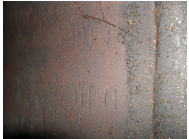
Photo 10: Fit-Up Marks in Can 1 South of Circ. Weld
