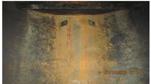
Photo 8: Corrosion on 0600 Position
