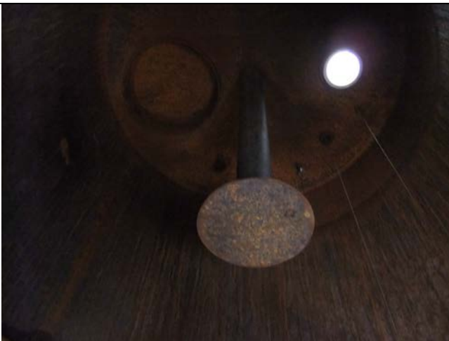
Photo 5 Description: Roof vent downcomer
