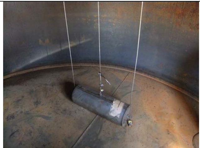
Photo 4 Description: Float with new cables
