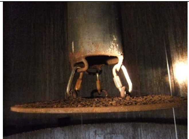
Photo 6 Description: Links holding baffle in place on roof vent downcomer
