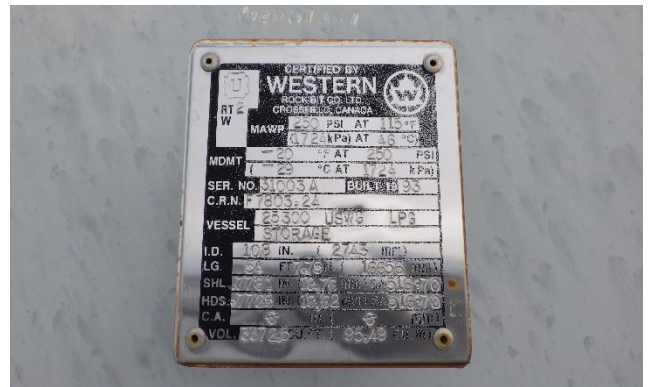
Photo 4 Description: Vessel Nameplate
