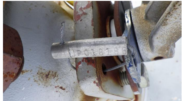
Photo 8 Description: PSV Valve Carsealed Open
