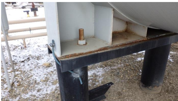
Photo 11 Description: Anchor Bolts/Ground
