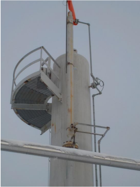
13 - T-500 GLYCOL CONTACTOR - E-503 GAS_GLYCOL EXCHANGER
