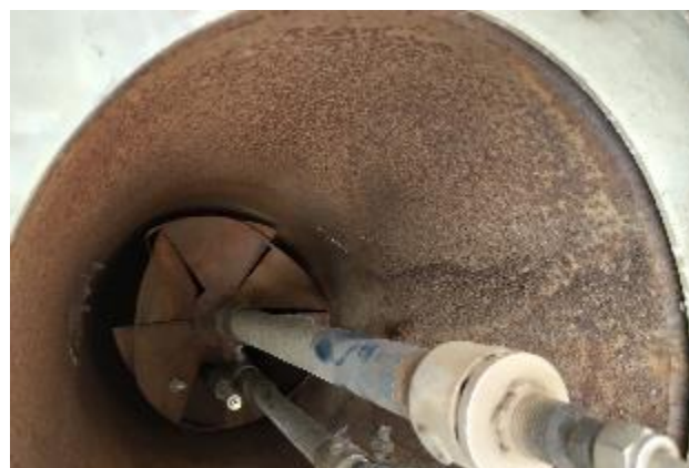
Photo 6 Description: Fire tube burner assembly.
