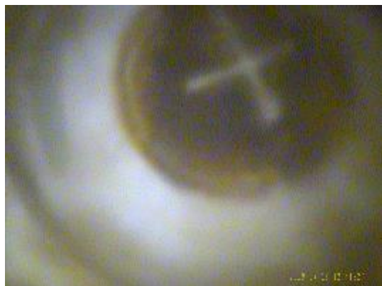
Photo 9 Description: Separator boot vortex breaker inside.
