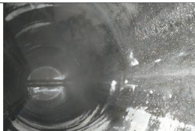
Photo 4 Description: Reboiler after clean up.
