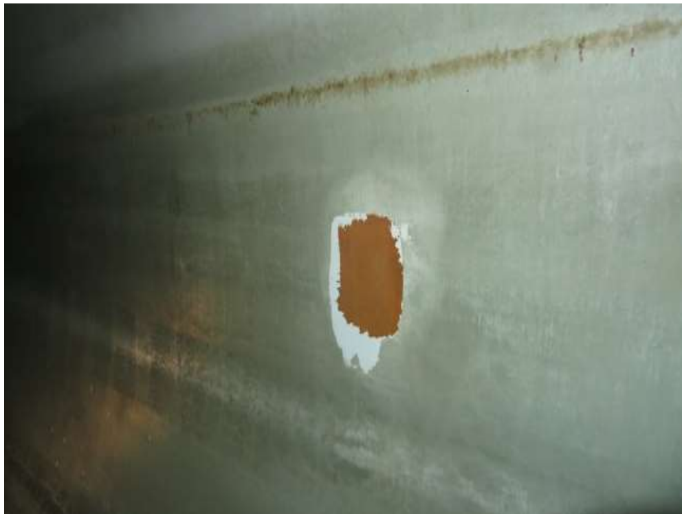
HISTORICAL COATING REPAIR
