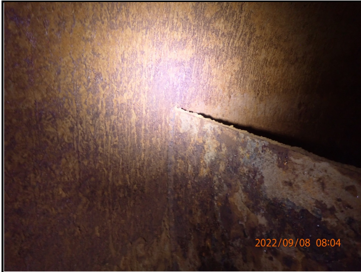
Wier to Shell Weld
