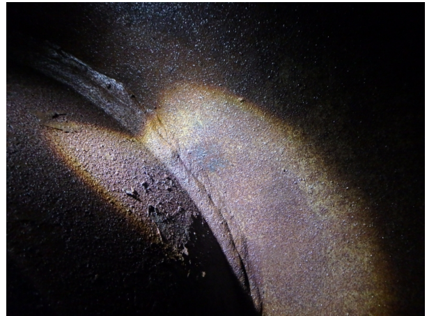
Photo 16: Internal Weld
