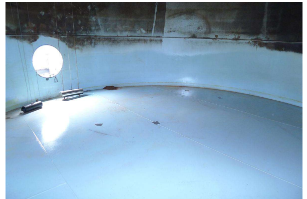
Internal shell/floor - note two level floats, one in front of manway
