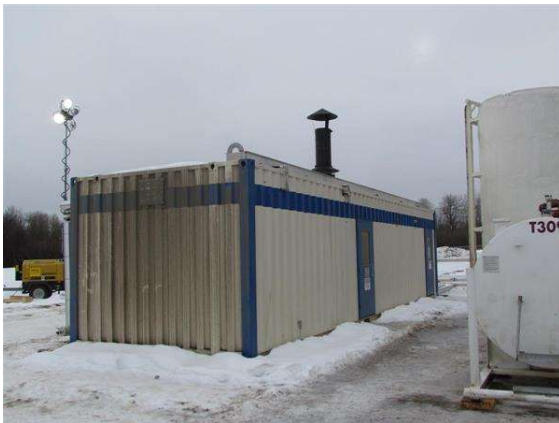
Building housing the boiler blowdown vessel
