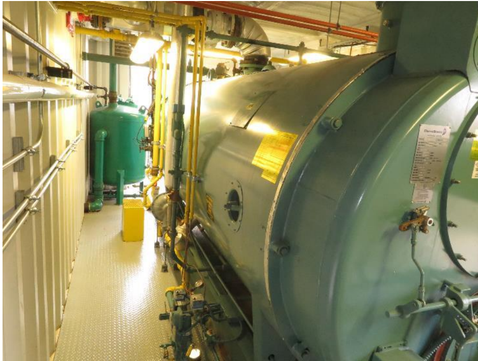
Cladding, base, and piping
