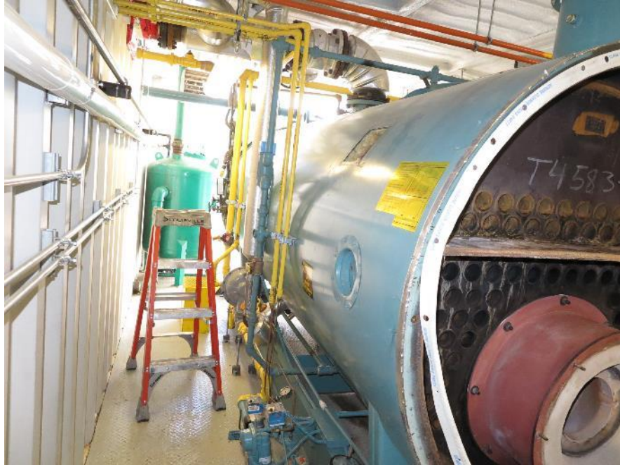
Cladding, base, and piping
