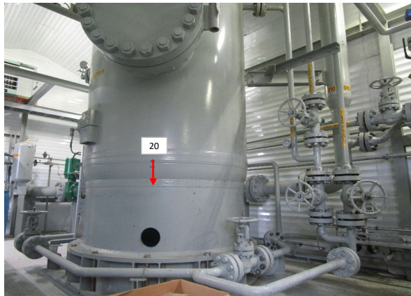
- TML 20 taken on bottom head of vessel
