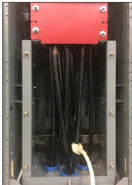
Figure 66 – First Cable Lacing Loop
