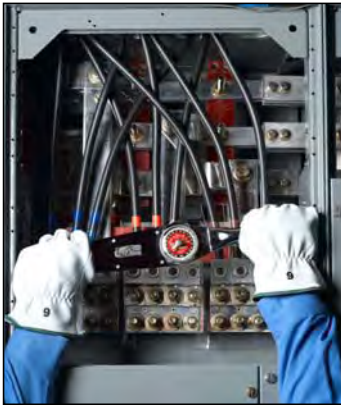
Figure 82 – Main Lug Compartment Torque Connection
