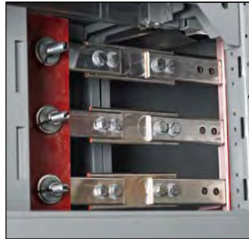
Figure 31 – Incorrect Application of Single-Bar Splice on Fork-Type Bus
