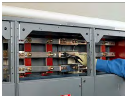
Figure 44 – 85,000 A Bracing Option
