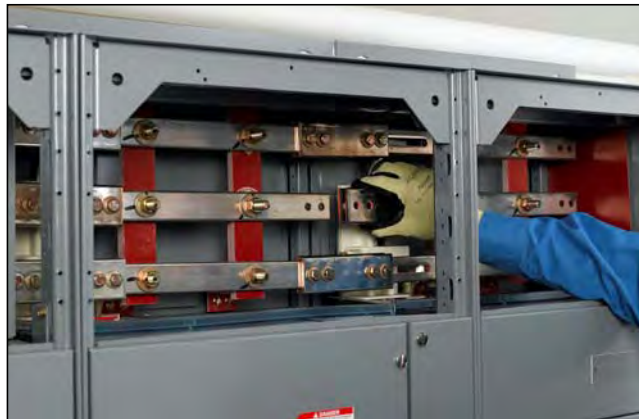
Figure 38 – Align the Splice and Bus Holes
