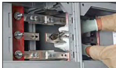
Figure 32 – Remove Bolts from Single-Splice Bar
