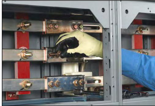
Figure 40 – Place a Conical Washer Under the Bolt Head
