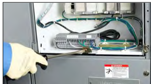
Figure 139 –Tightening the Control Unit Lock-in Panel (when supplied)
