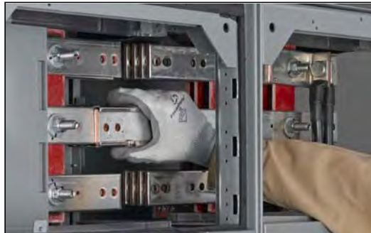
Figure 54 – Align the Splice and Bus Holes
