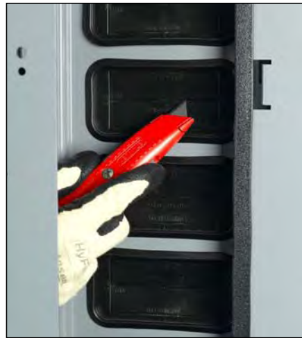
Figure 135 –Cutting the Vertical Wire Trough Grommet (when supplied)
