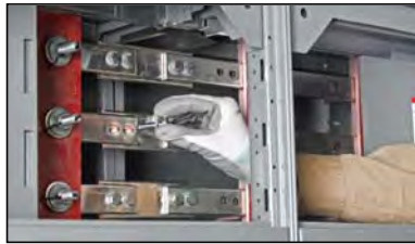
Figure 35 – Place a Conical Washer Under the Bolt Head
