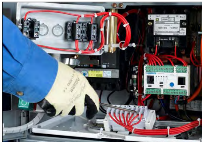
Figure 79 – Pull-apart Type Terminal Blocks
