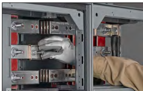
Figure 55 – Insertion de boulons de raccordement
