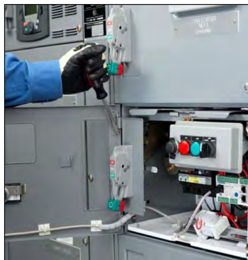
Figure 100 –Driving Out Hinge Pin
