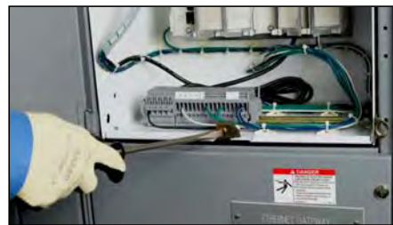
Figure 92 – Releasing the Lock-in Device (when supplied)
