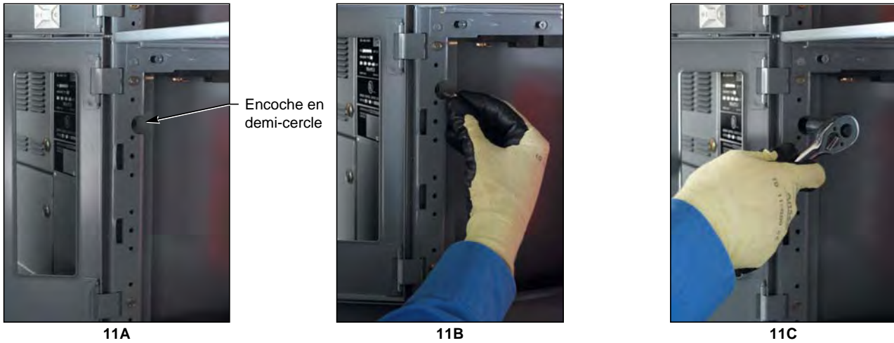
Figure 11 – Boulonnage des sections ensemble
