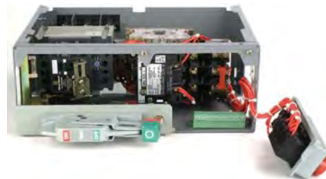
Figure 103 –Control Station Plate Removed
