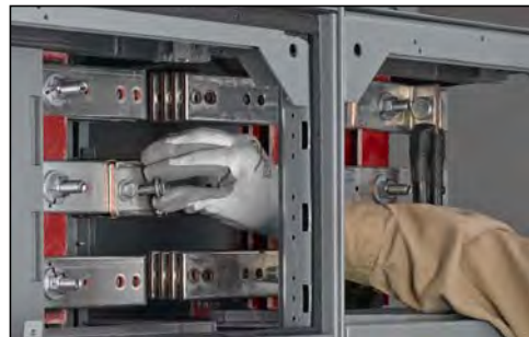
Figure 55 – Insert the Splice Bolts
