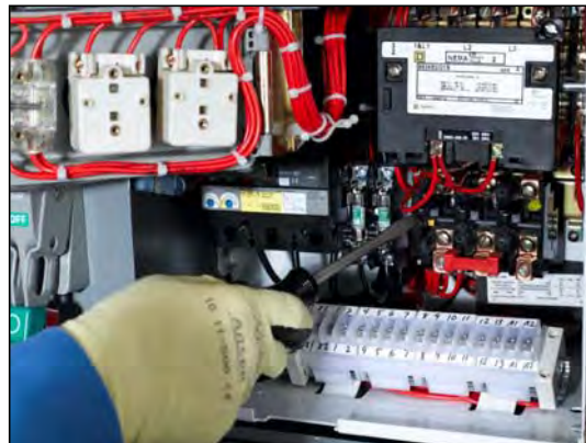
Figure 110 –Tripping the Overload Relay
