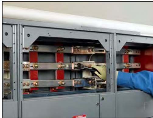
Figure 37 – Remove the Left Bolts and Loosen the Right Bolts on the Splice Assembly
