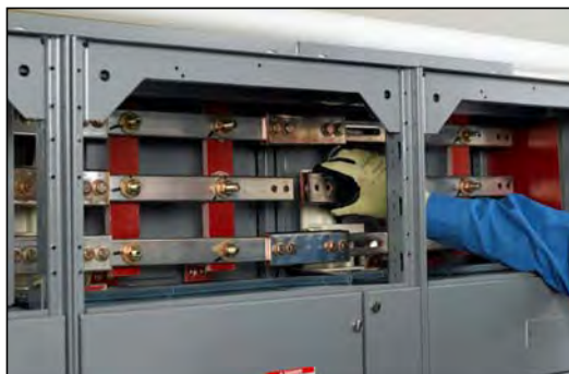
Figure 45 – Slide the Splice Assembly to the Left
