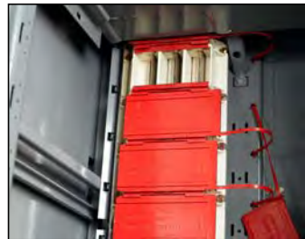
Figure 136 –Removing the Manual Bus Shutter
