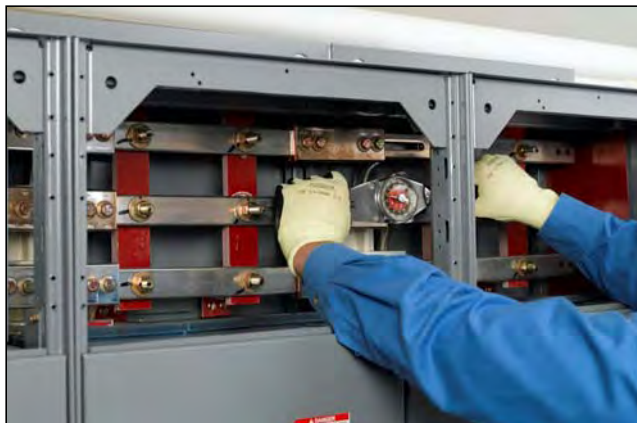
Figure 41 – Torque the Bolts
