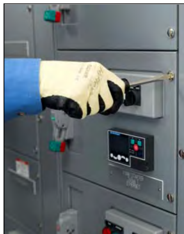
Figure 102 –Loosening Captive Fasteners
