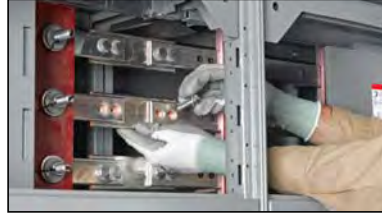
Figure 33 – Move and Align the Splice Bar to the Bus Holes
