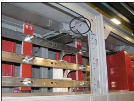
11F: Top Front Side Channel Connection
