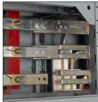
Figure 31 – Incorrect Application of Single-Bar Splice on Fork-Type Bus
