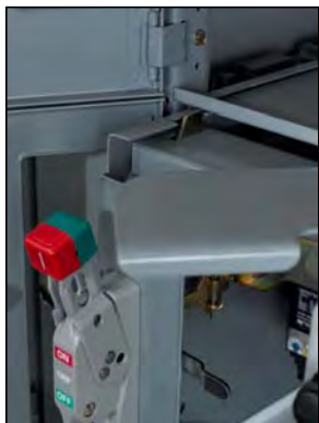
Figure 96 – Operating the Mechanism-to-Structure Interlock
