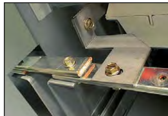
Figure 50 – Ground Bar Bolt Replaced
