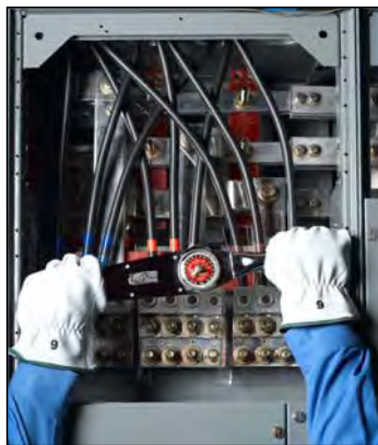
Figure 87 – Main Lug Compartment Torque Connection
