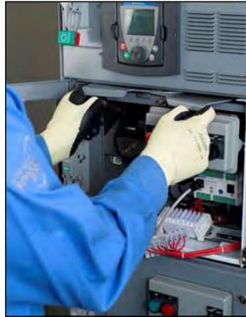
Figure 137 –Engaging the Cam Mechanism
