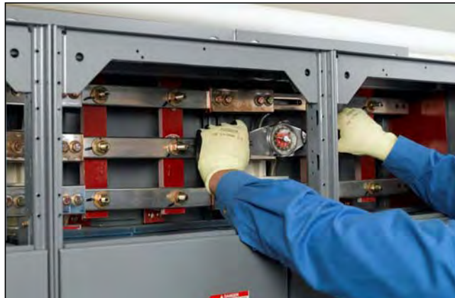
Figure 48 – Torque All Bolts
