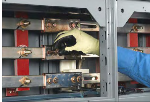
Figure 47 – Place a Conical Washer Under the Bolt Head
