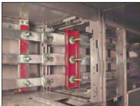
Figure 44 – 85,000 A Bracing Option
