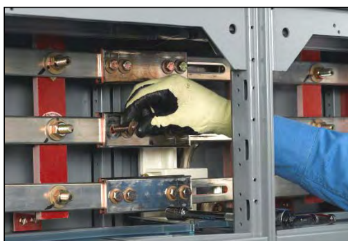
Figure 46 – Insertion de boulons de raccordement
