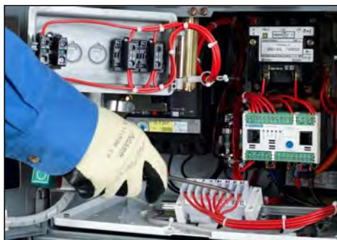
Figure 143 –Connecting Control Leads to the Terminal Blocks
