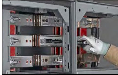
Figure 53 – Remove the Bolts from the Splice Assembly
