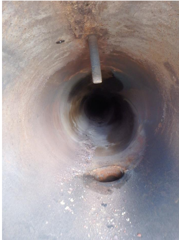
Figure 5: Firetube Internal Overview
