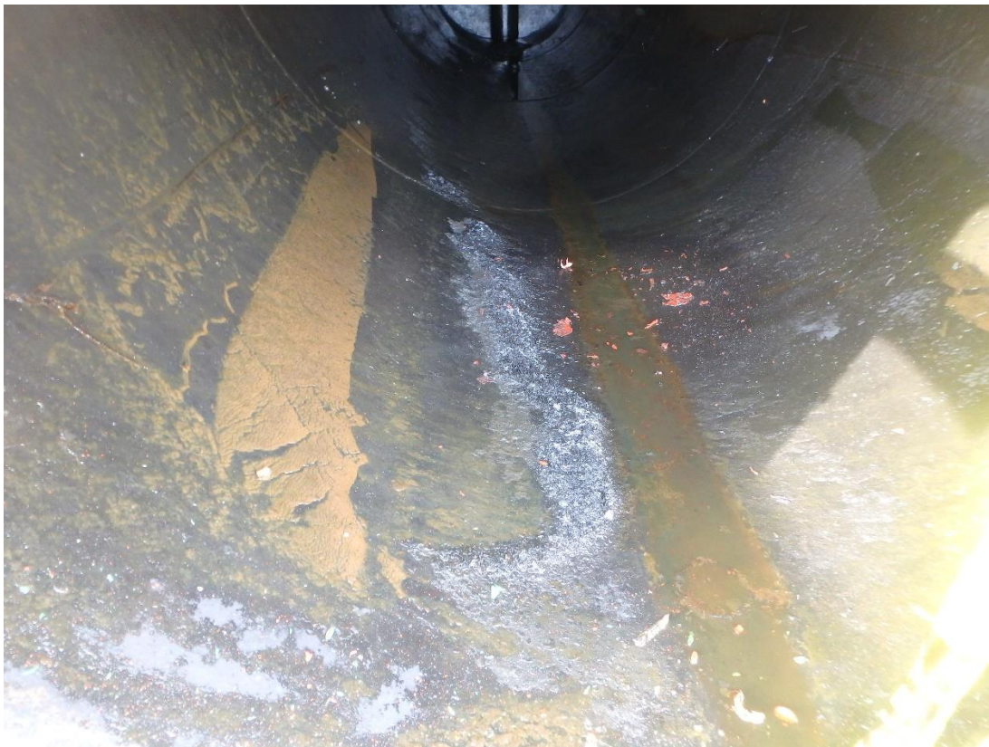
Figure 2: Reboiler Lower Shell Overview
