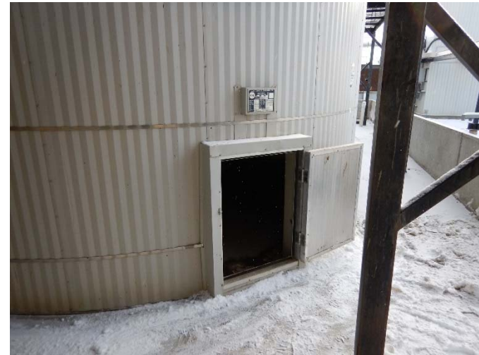
Bottom of Tank Entrance
