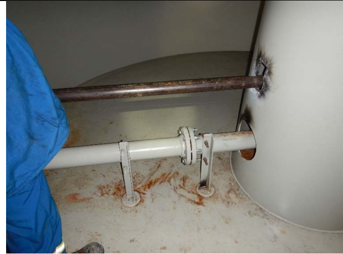
Tank Bottom Cone Drain
