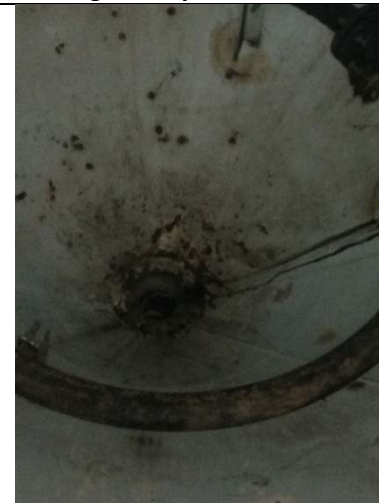
Coating Holidays on Cone Bottom
