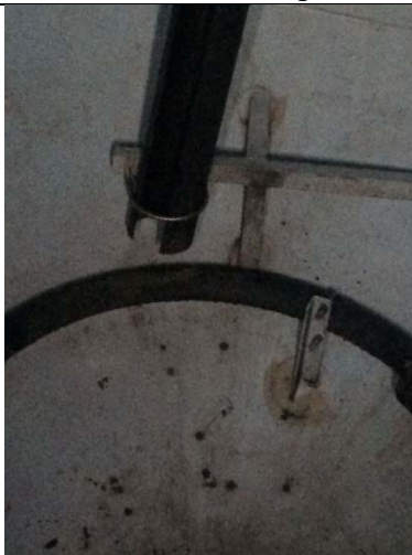
Coating Holidays on Cone Bottom
