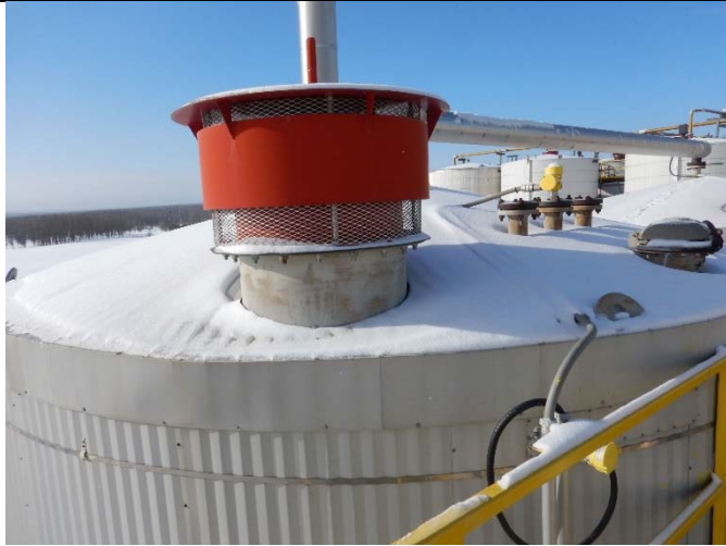
Tank Roof Overview
