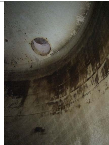
Tank Roof and Shell Interface
