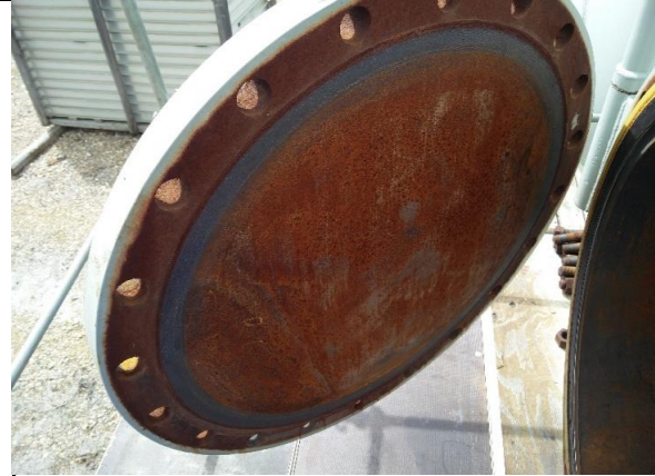
Photo 8 Description: Manway blind slight surface rust
