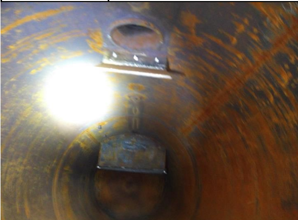
Photo 9 Description: Internal inspection, slight surface rust
