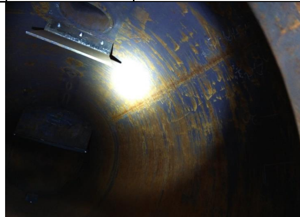
Photo 12 Description: Internal inspection, slight surface rust
