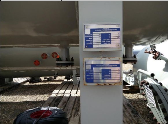
Photo 3 Description: 2 nameplates, 1 metric and 1 SAE
