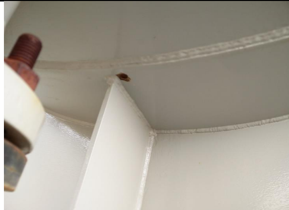
Photo 16 Description: Saddle weep hole still with grease
