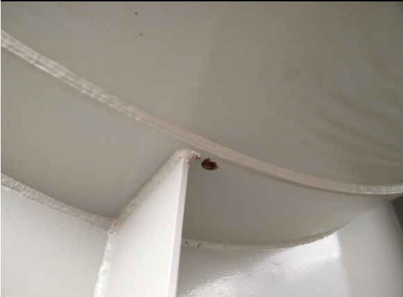
Photo 15 Description: Saddle weep hole still with grease
