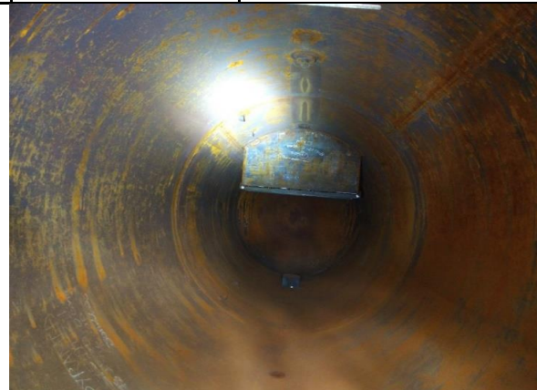
Photo 10 Description: Internal inspection, slight surface rust
