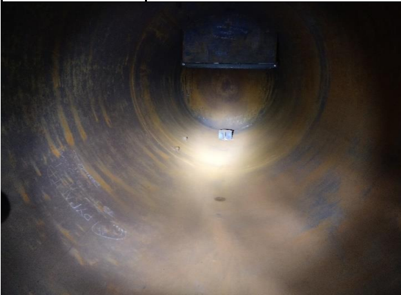
Photo 11 Description: Internal inspection, slight surface rust
