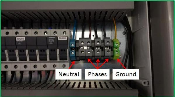
The three-phase connection for the consumption of the ORC is made by an electrical wire G5 (3 phases, ground and neutral). The section must be 6 mm². The distance between the ORC and the connection point must be adapted to this section, regarding the maximum 5 kW consumption.
