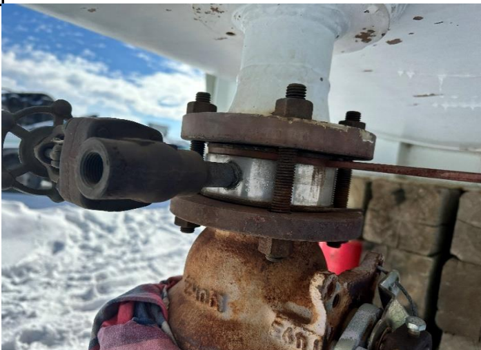
Photo 6: Bled ring and valve installed
