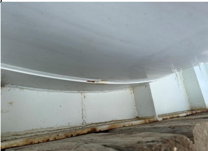
Photo 4: Saddles with vent in welding
