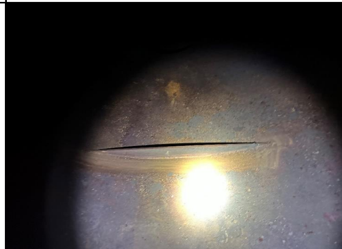
Photo 4: Weir Plate in good condition
