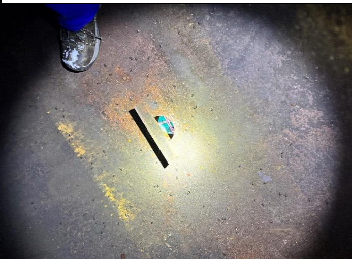
Photo 5: Vortex Breaker in good condition
