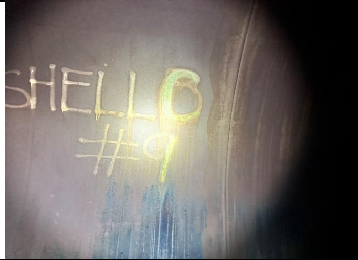
Photo 2: Shell longseam and circseam welding in good condition
