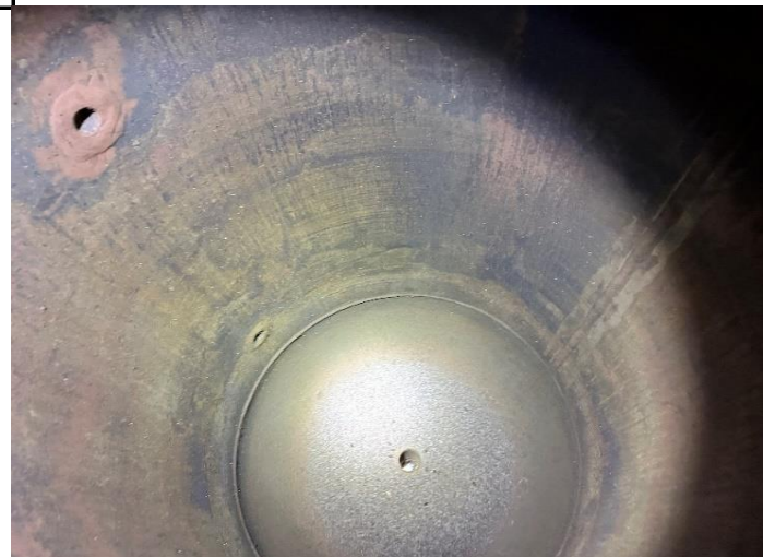
Photo 6: Sump in good condition, to be cleaned of debris
