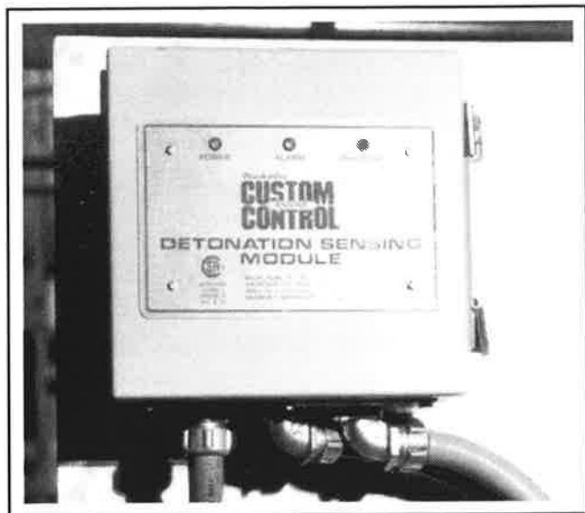
Figure 1.10-4. CEC Detonation Sensing Module
