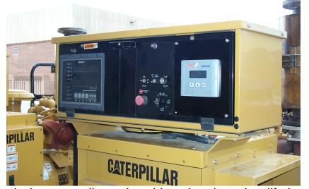
reductions in exhaust gas pollutants, particularly Oxides of Nitrogen (NOx), Carbon Monoxide (CO), and Hydrocarbons (HC). Catalytic converters require a constant air fuel ratio to the engine in order to work effectively – the *EDGE* provides the precise control needed to maintain that constant air fuel ratio. The resulting system provides accurate and stable control, which results in high catalyst efficiencies and reduced stack emissions. By automatically maintaining an optimum air fuel mixture,
