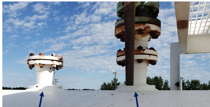
UT 16 4" Nozzel with Repad No Inspection UT 17 4" Nozzel with Repad No Inspection
