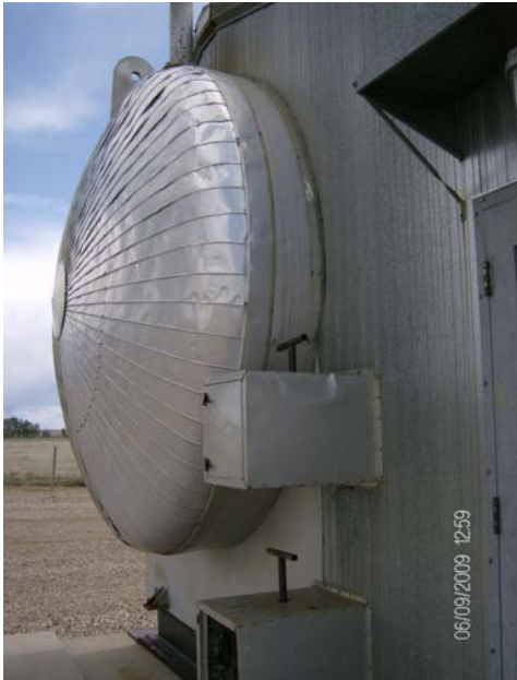
Grand Forks-FWKO_ Outside Bldg.
