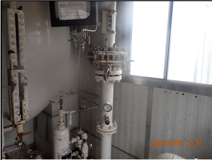
Meter Run Piping
