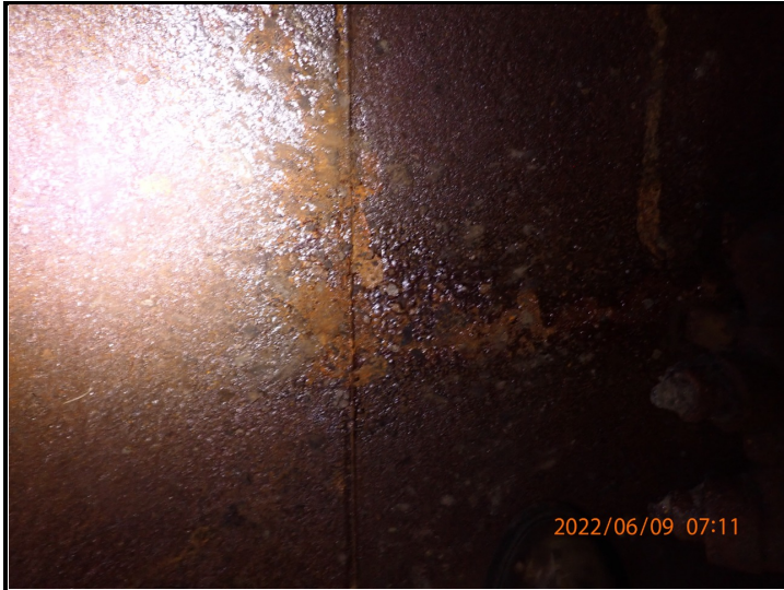
Head to Shell Weld
