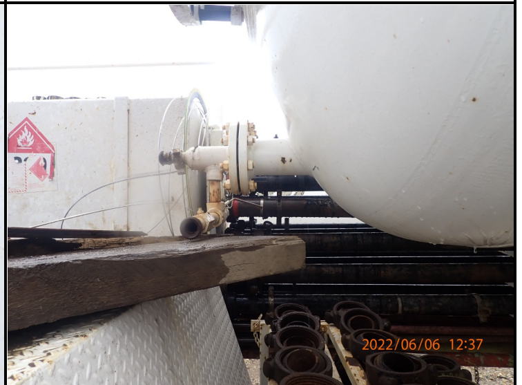
Sparging and Coil Connections
