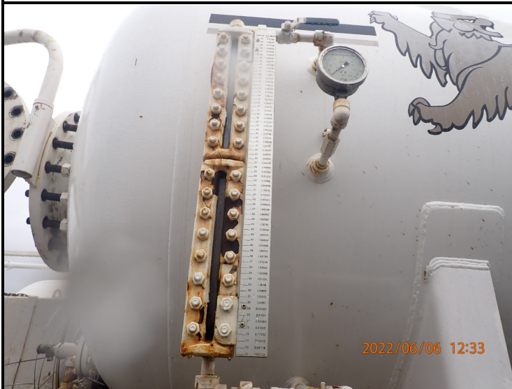
Coil Inlet and Level Gauge
