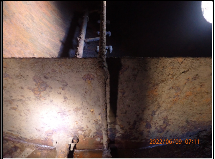
Weir and Pipe Penetrations
