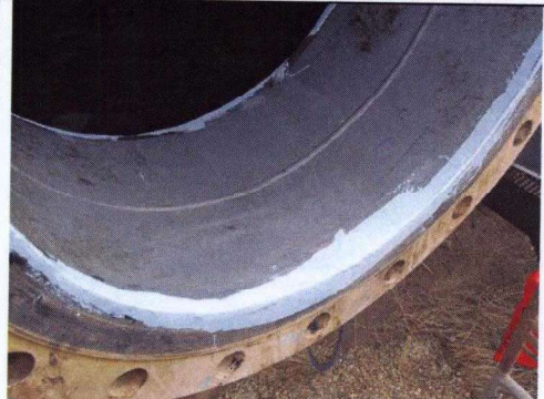
Man Way patch coating
