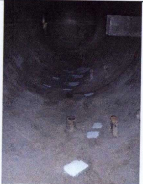
Patches coated after repair
