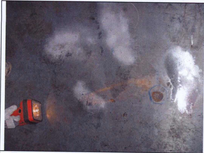
Five repairs tested, shell section 2 south of manway
