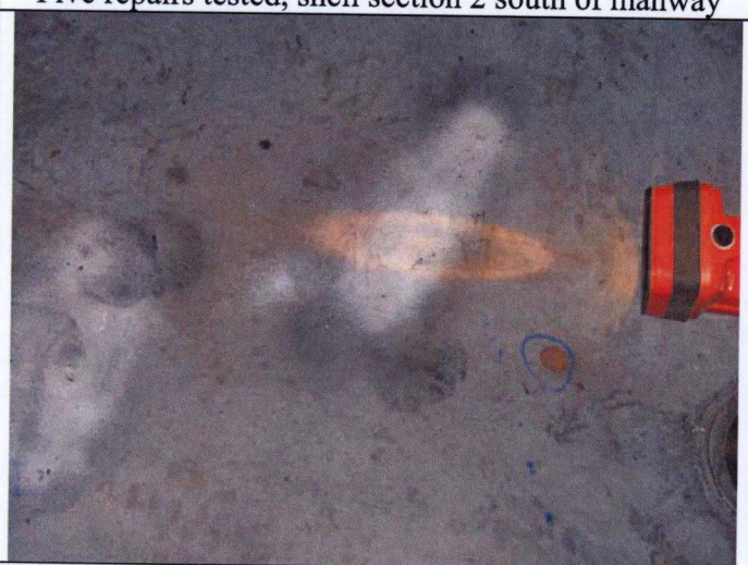
Two repairs tested, shell section 3 south of manway
