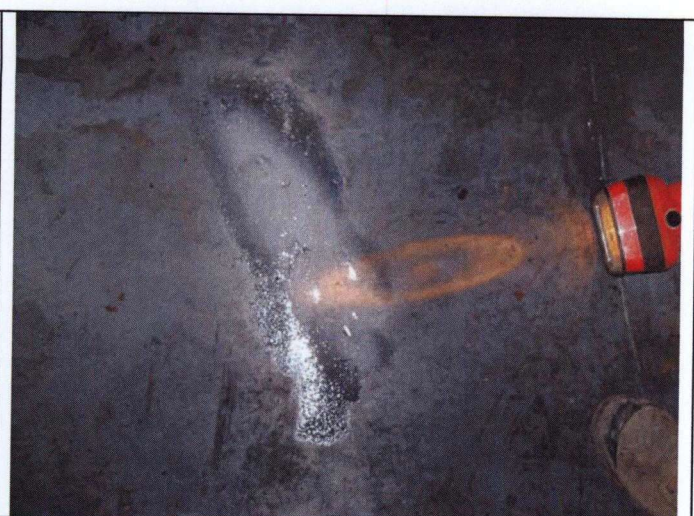
Two repairs tested, shell section 2 south of manway
