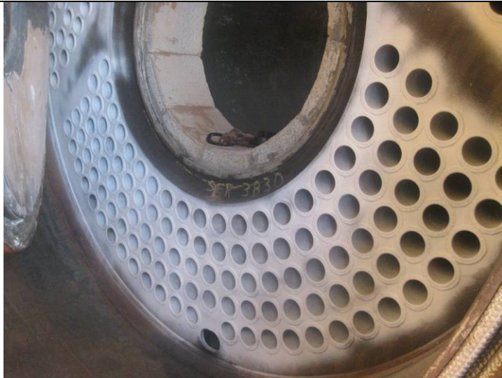
View of areas inspected in bottom of Burner End.
