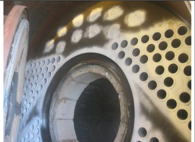
View of areas inspected in top of Burner End.
