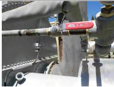
Main burner test firing valve
