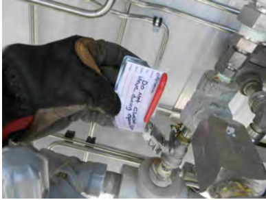
Isolation valve on pressure switch (PSLL)
