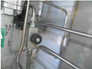
Speed control valve for SSV
