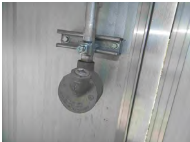
Hazardous area conduit seal at the wall
