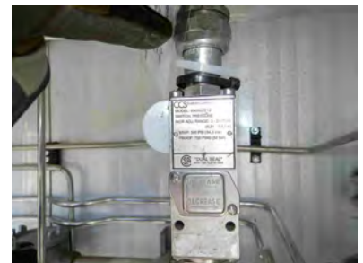
PSHH - High pressure shutdown
