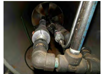
Main burner and pilot close-up
