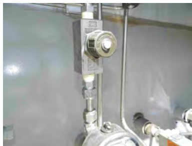
Speed control valve for FCV
