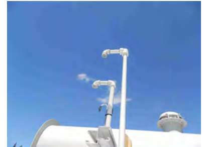
Vent line terminations
