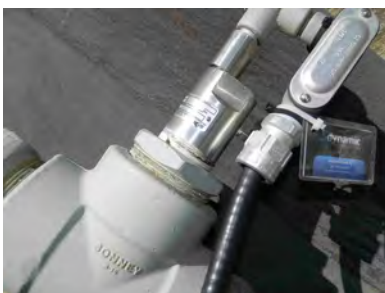
LSLL - Low bath fluid shutdown
