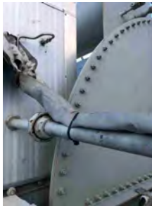
Pilot fuel train tied with main fuel train for support
