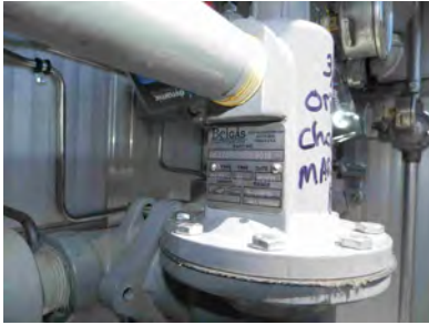
Main fuel train pressure regulator - PRV
