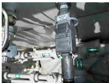
TSHH - High temperature shutdown
