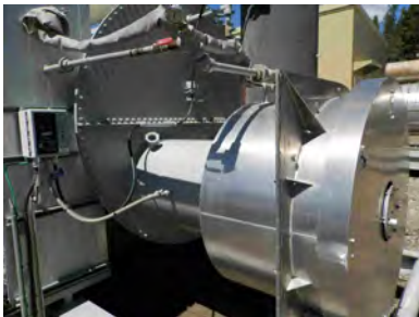
Pilot fuel train outside enclosure not supported (NON-CONFORMANCE)
