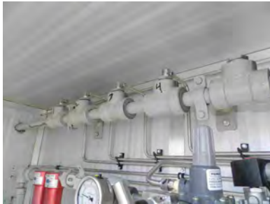
Vent line terminations,Vent lines
