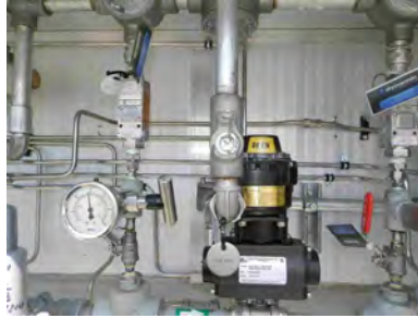
Main fuel train safety shut-off valve - SSV
