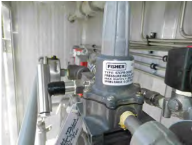
Pilot pressure regulator - PRV
