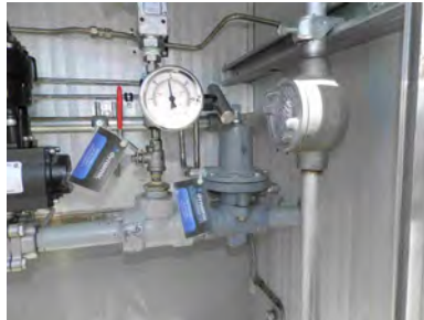
FCV - Main flow control valve
