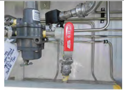
Pilot manual fuel shut-off valve
