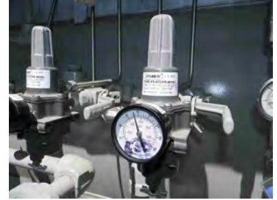
Instrument gas regulator (PRV) to SSV
