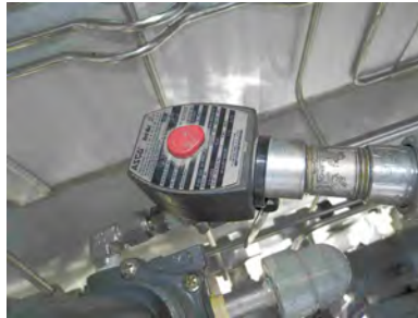
Pilot safety shut-off valve - SSV
