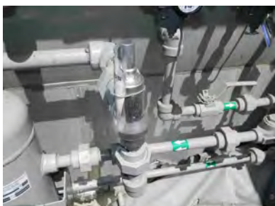
Upstream overpressure protection - PSV
