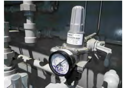
Instrument gas regulator (PRV) to FCV
