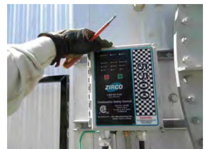
Burner Management System - BMS
