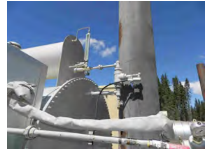
Pilot fuel train not supported (NON-CONFORMANCE)
