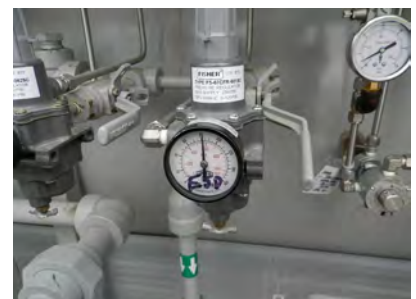
Instrument gas regulator (PRV) to SSV
