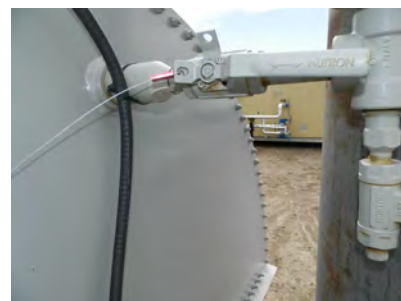
Isolation valve on LSLL
