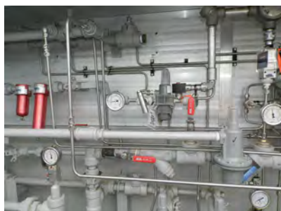
Pilot manual fuel shut-off valve
