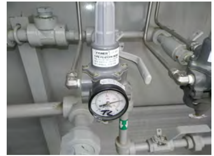
Instrument gas regulator (PRV) to FCV
