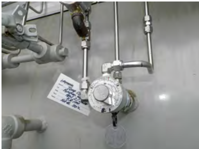
TC - pneumatic process temperature control
