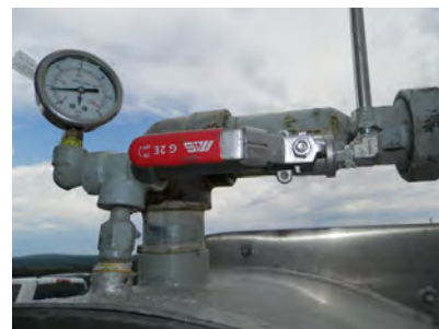
Pilot burner test firing valve
