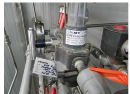
Pilot pressure regulator - PRV
