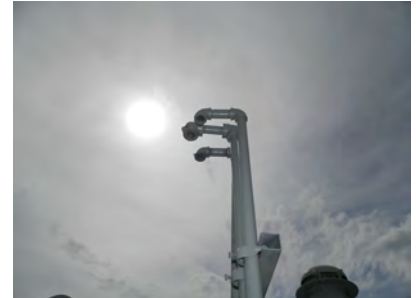
Vent line terminations
