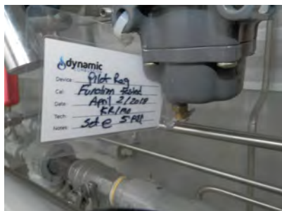
Pilot PRV pressure calibration tag
