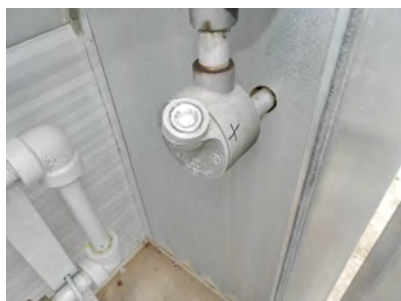
Hazardous area conduit seal at the wall
