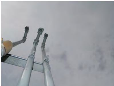
Vent line terminations
