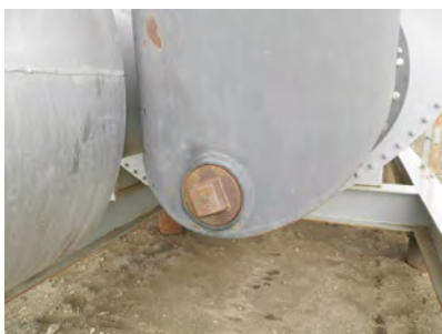
Stack cleanout / access port
