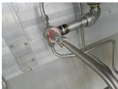
SSV 3-way solenoid valve (NON-CONFORMANCE)
