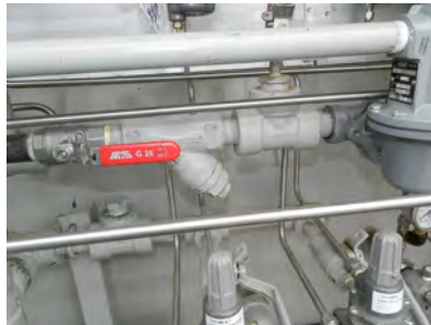
Manual shut-off valve and Y-strainer
