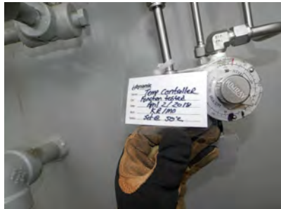
TC - pneumatic process temperature control calibration tag
