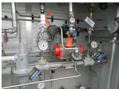
Main fuel train safety shut-off valve - SSV (NON-CONFORMANCE)
