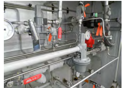
Main fuel train pressure regulator - PRV
