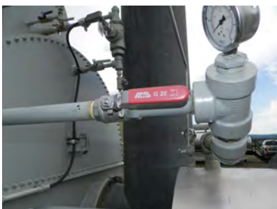
Main burner test firing valve
