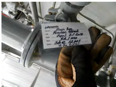
Main PRV pressure calibration tag
