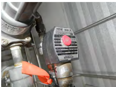
Pilot safety shut-off valve - SSV
