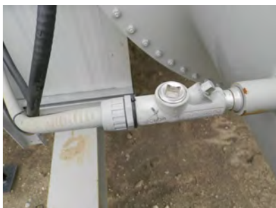
Hazardous area electric seal at the windbox
