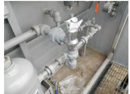
Upstream overpressure protection - PSV
