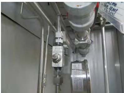
Speed control valve for main FCV
