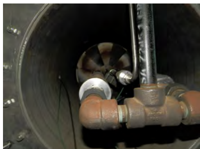
Main burners and pilot close-up
