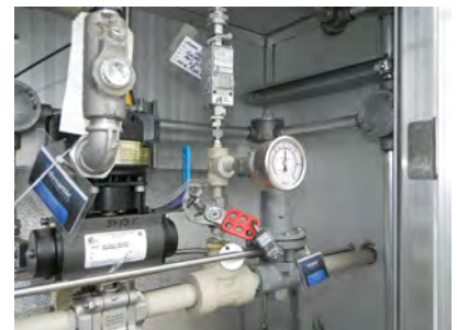
PSHH - High pressure shutdown
