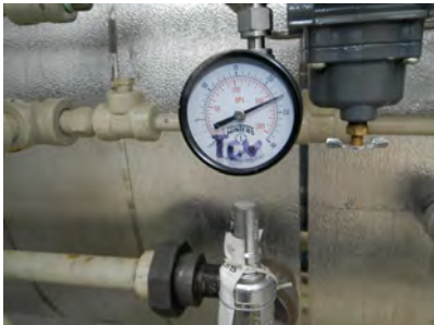
Instrument gas regulator (PRV) to FCV pressure gauge
