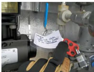
Isolation valve on pressure switch (PSHH)
