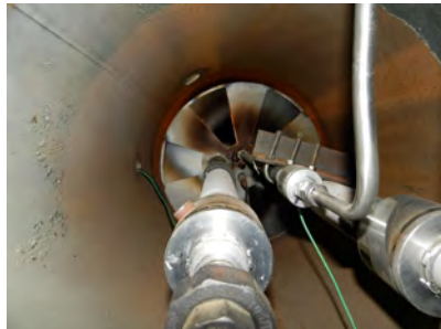
Main burners and pilot close-up
