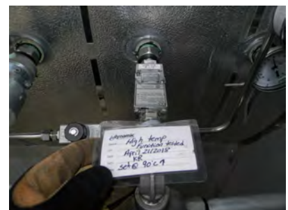
TSHH - High temperature shutdown calibration tag
