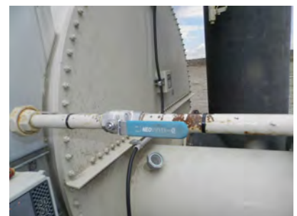
Main burner test firing valve
