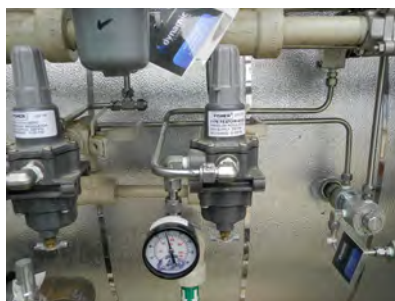
Instrument gas regulator (PRV) to SSV
