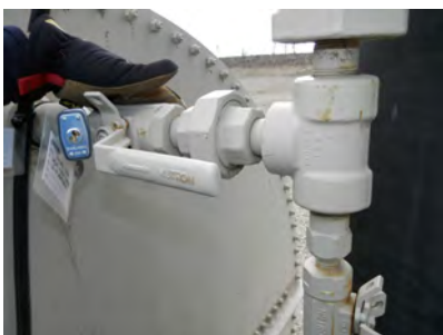
Isolation valve on LSLL
