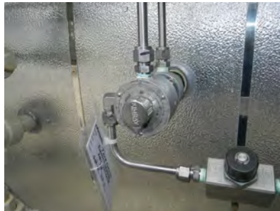
TC - pneumatic process temperature control
