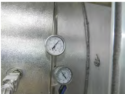
Bath fluid temperature gauge
