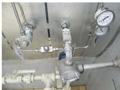
TSHH - High temperature shutdown
