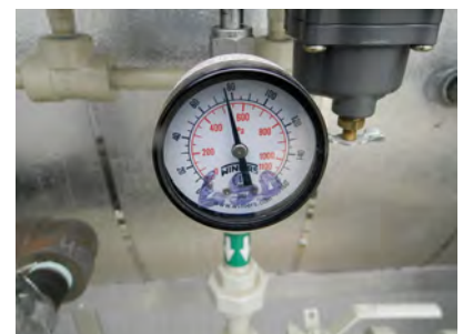
Instrument gas regulator (PRV) to SSV pressure gauge
