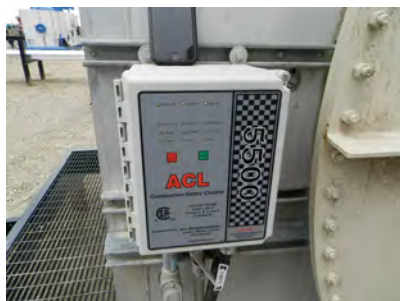
Burner Management System - BMS
