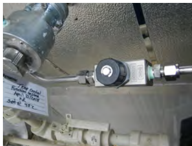
Speed control valve for main FCV
