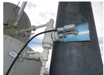
LSLL - Low bath fluid shutdown
