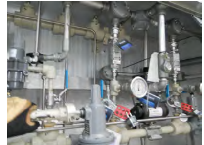
PSLL - Low pressure shutdown
