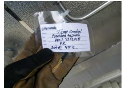
TC - pneumatic process temperature control calibration tag
