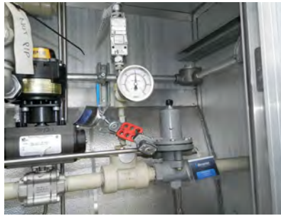
FCV - Main flow control valve
