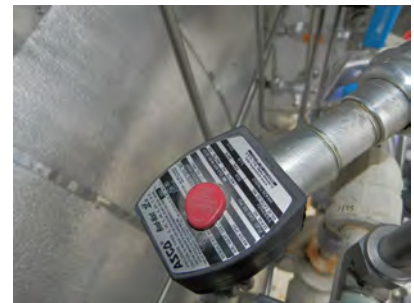
Pilot safety shut-off valve - SSV
