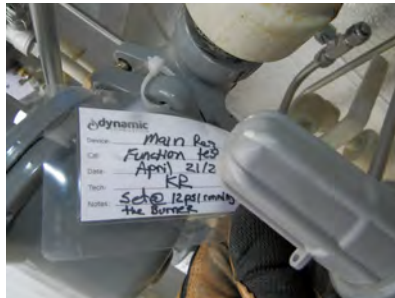
Main PRV pressure calibration tag
