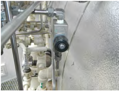
Speed control valve for main SSV
