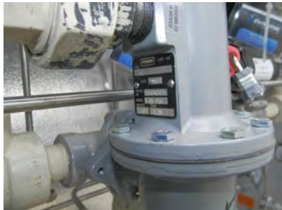
Main fuel train pressure regulator - PRV
