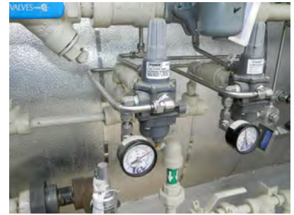
Instrument gas regulator (PRV) to FCV
