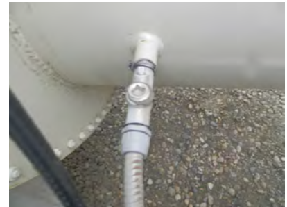
Hazardous area electric seal at the windbox
