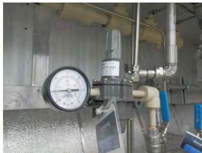
Pilot pressure regulator - PRV
