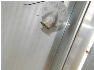
Hazardous area conduit seal at the wall
