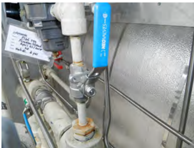
Pilot manual fuel shut-off valve
