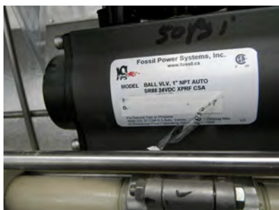
Main fuel train safety shut-off valve - SSV
