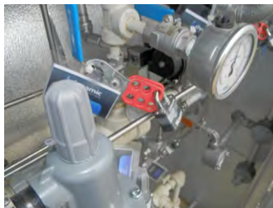
Isolation valve on pressure switch (PSLL)
