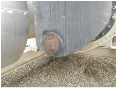
Stack cleanout / access port
