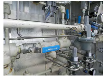
Manual shut-off valve and Y-strainer
