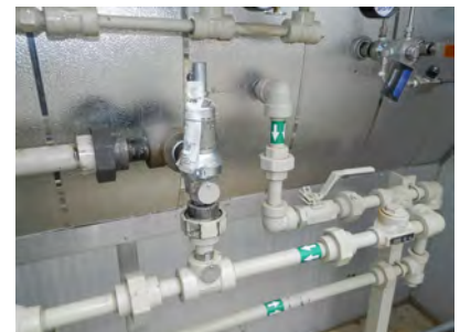
Main fuel train overpressure protection - PSV
