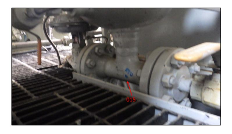
MPI on Category D welds completed and areas inspected did not exhibit any relevant defects or indications at time of inspection.AJB
