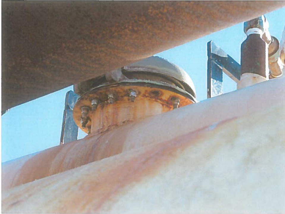
Flame Burner Gasket is broken.
